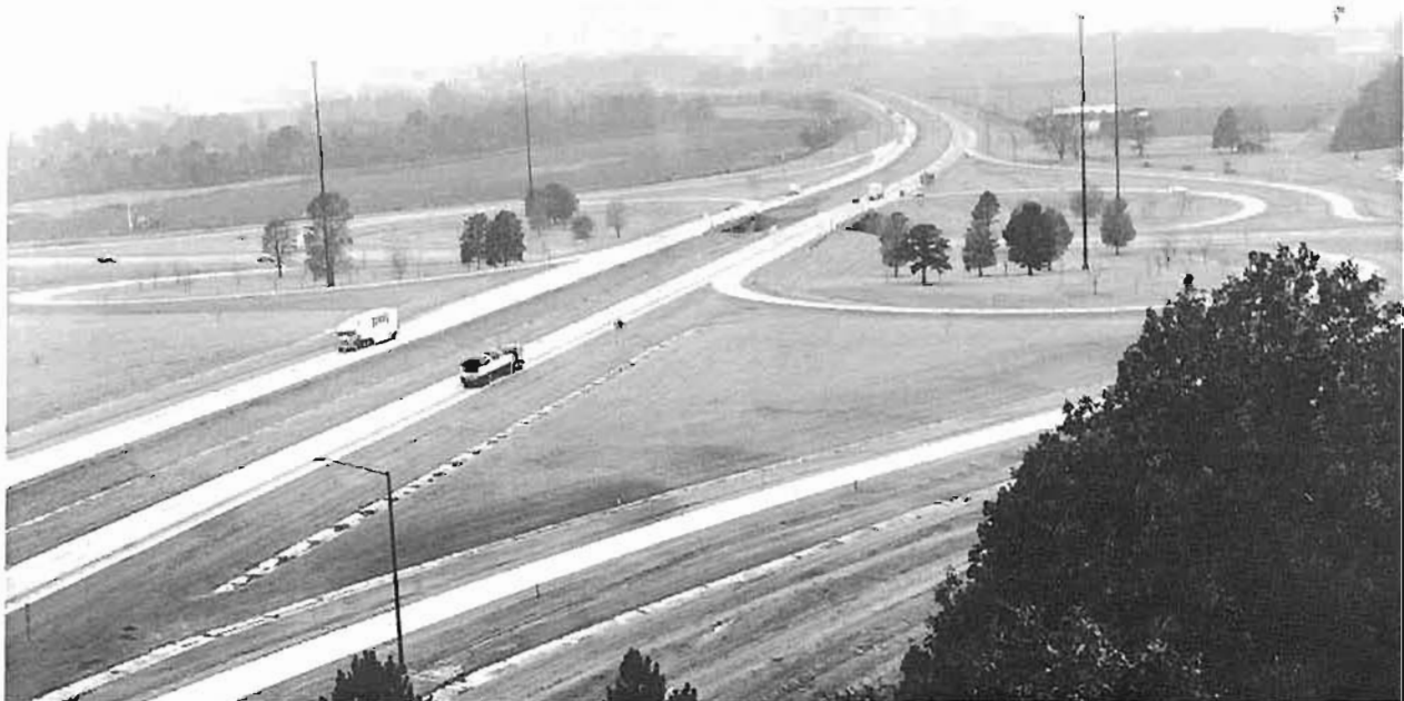
The Highway 1-Interstate 40 Interchange at Forrest City sports new high mast lights
